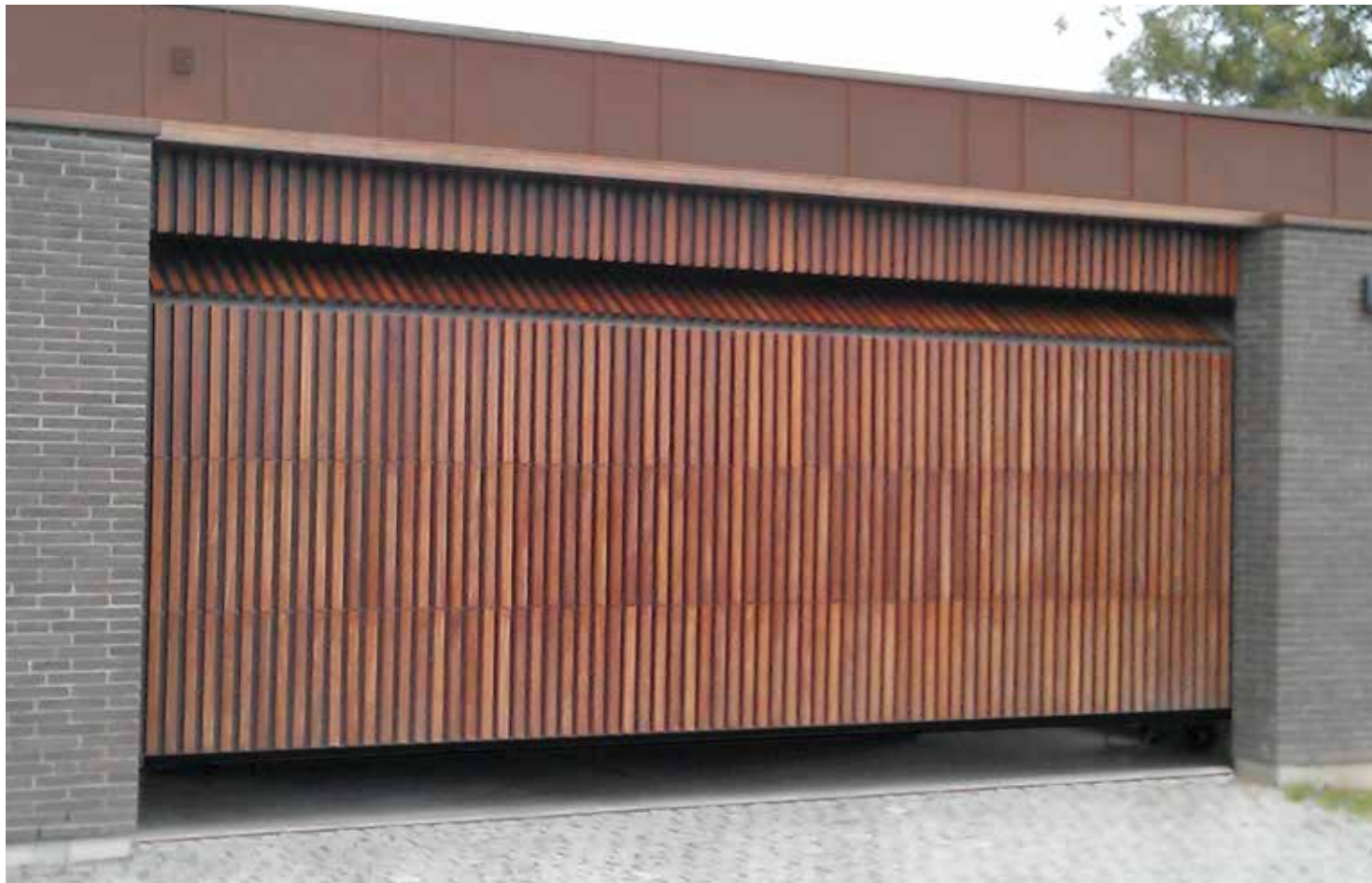
Garage door and fascia panel clad with 50x50 mm larch scantlings.
