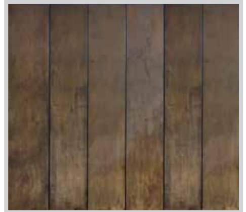
Side-sliding door clad with corten panels.
