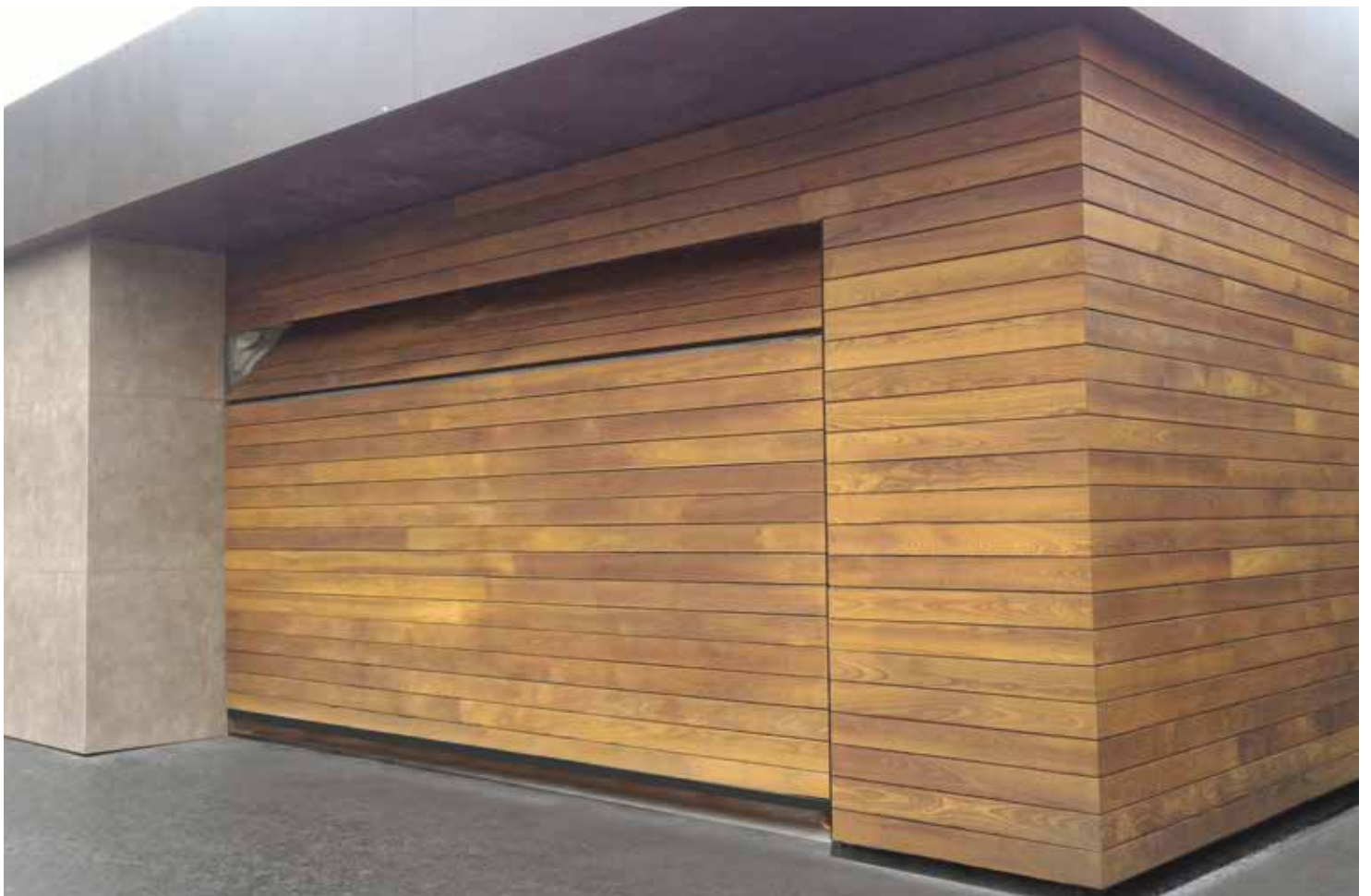
Facade-flush garage door clad with oak planks same as part of house facade to get 'concealed' door effect.
